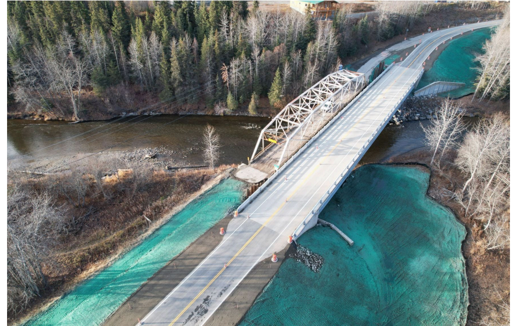
Anchor River Bridge Replacement Project, 2021-2022
