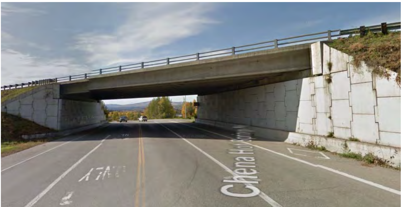
Figure 1: Similar structure Steese Highway over Chena Hot Springs Road, looking West.
