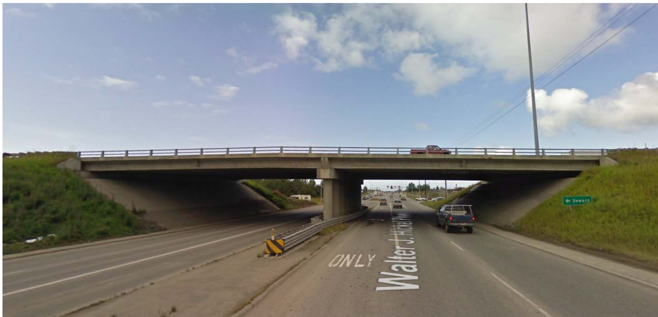
Figure 3: Similar structure Seward Highway over O'Malley Road, looking East.
