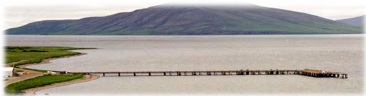
False Pass dock. Photo courtesy of DCRA.
