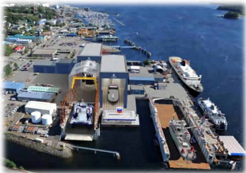
An aerial photo of the Alaska Ship and Drydock in Ketchikan. Photo from Vigor Industrial website.
